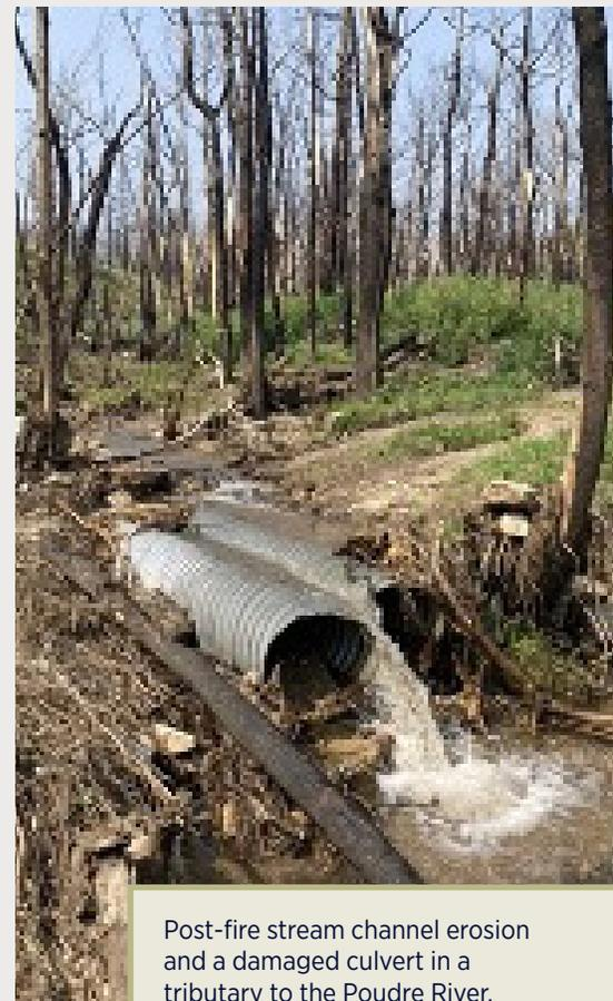
Post-fire stream channel erosion and a damaged culvert in a tributary to the Poudre River.
